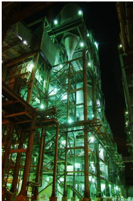
Calcination plant at Alumina Refinery of NALCO, after 2nd phase expansion.
