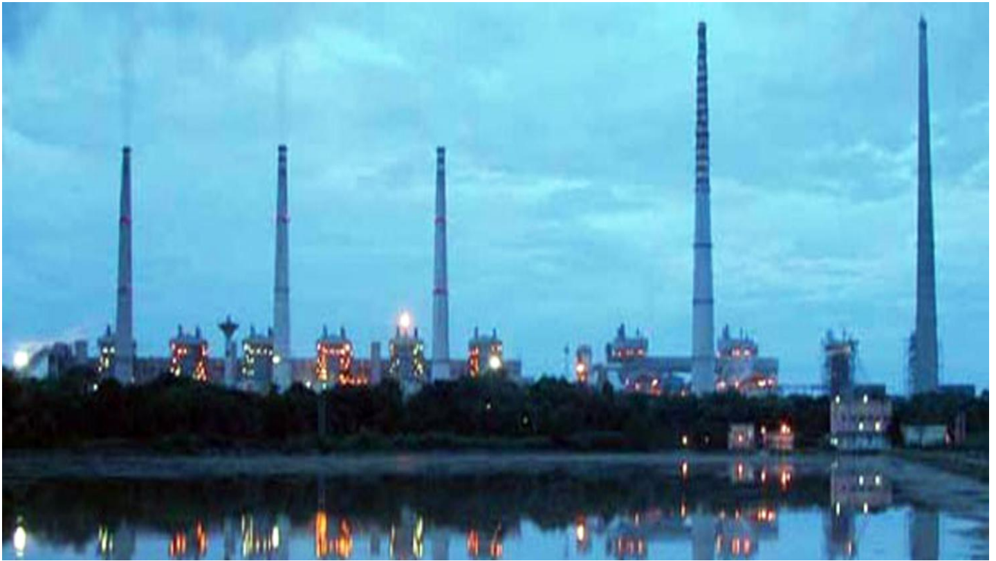
Captive Power Plant of NALCO
